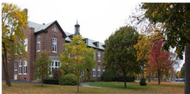
Stormonth Elementary School 7301 N. Longacre Road, Fox Point
